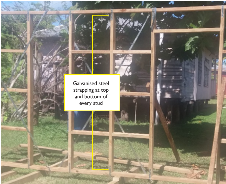
Figure A14: Stud wall frame with galvanised steel cyclone strapping (Source: Fiji Rural Housing Unit)
